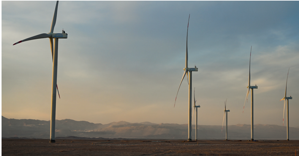
Engie Energia Chile S.A. (Chile)
